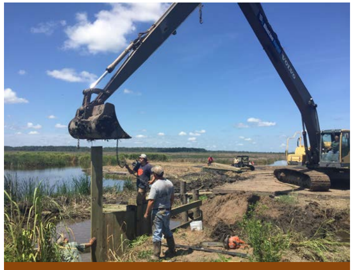
Construction of cross dike and installation of rice trunk to manage water levels for Black Rail. Nemours Wildlife Foundation
