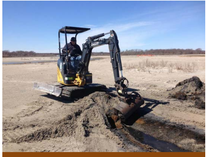
Thin layer deposition is a priority action in New York to help raise marshes from impacts of sea level rise. Wenley Ferguson, Save the Bay
