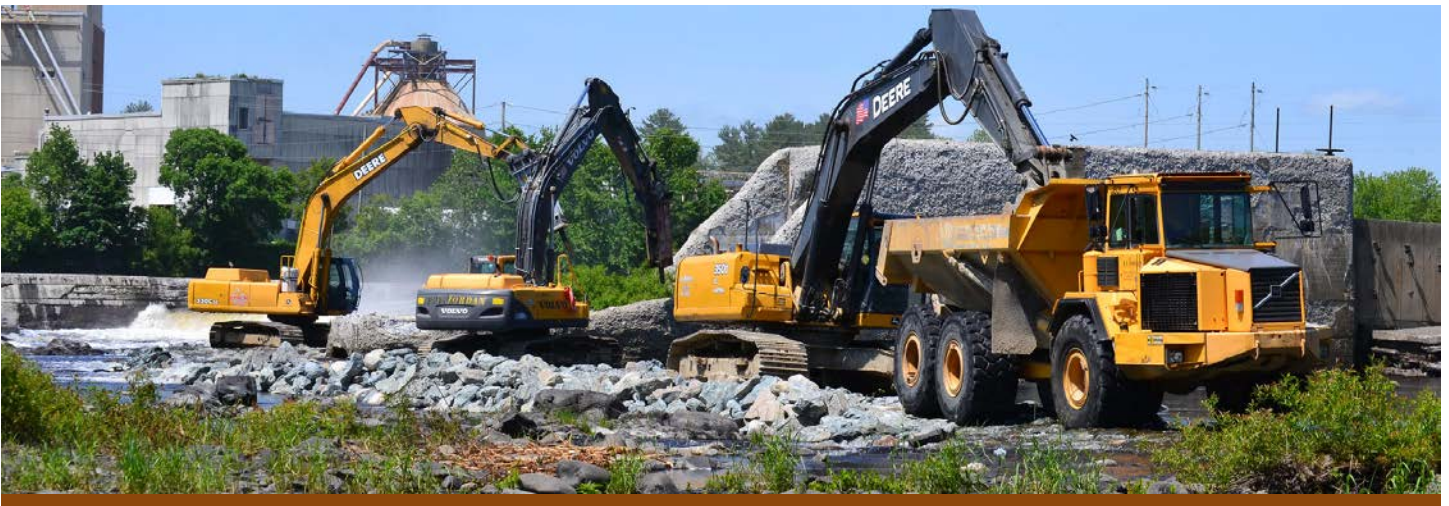
Restoring rivers by removing dams helps return the natural flow of sediments to rivers and estuaries. USFWS
