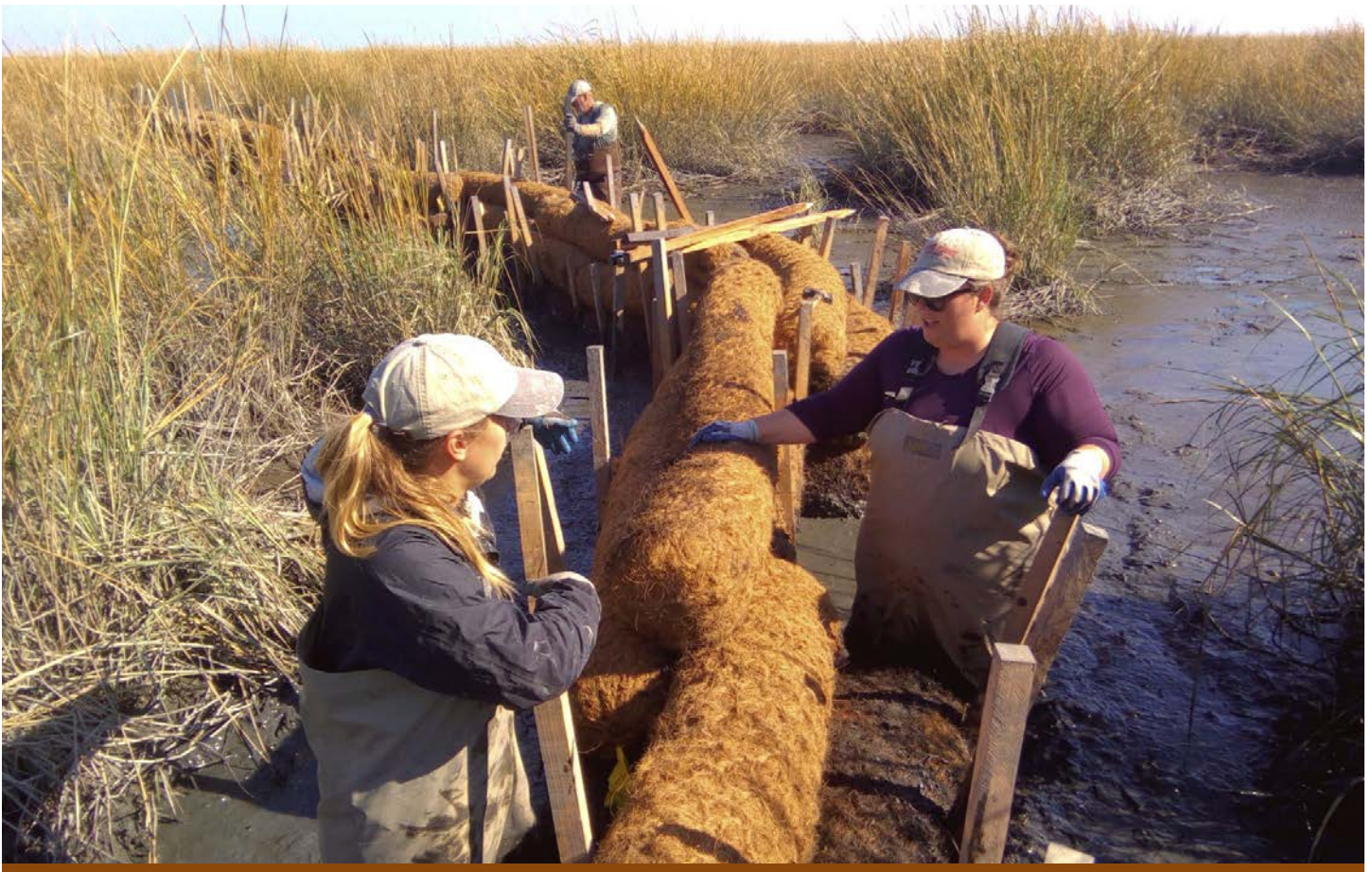
To offset elevation loss caused by salt hay farming, employees from American Littoral Society and Wildlife Restoration Partnerships construct a boundary with coconut coir logs to contain dredge material that will increase elevations to levels that can support the recovery of salt marsh. Shane Godshall.
